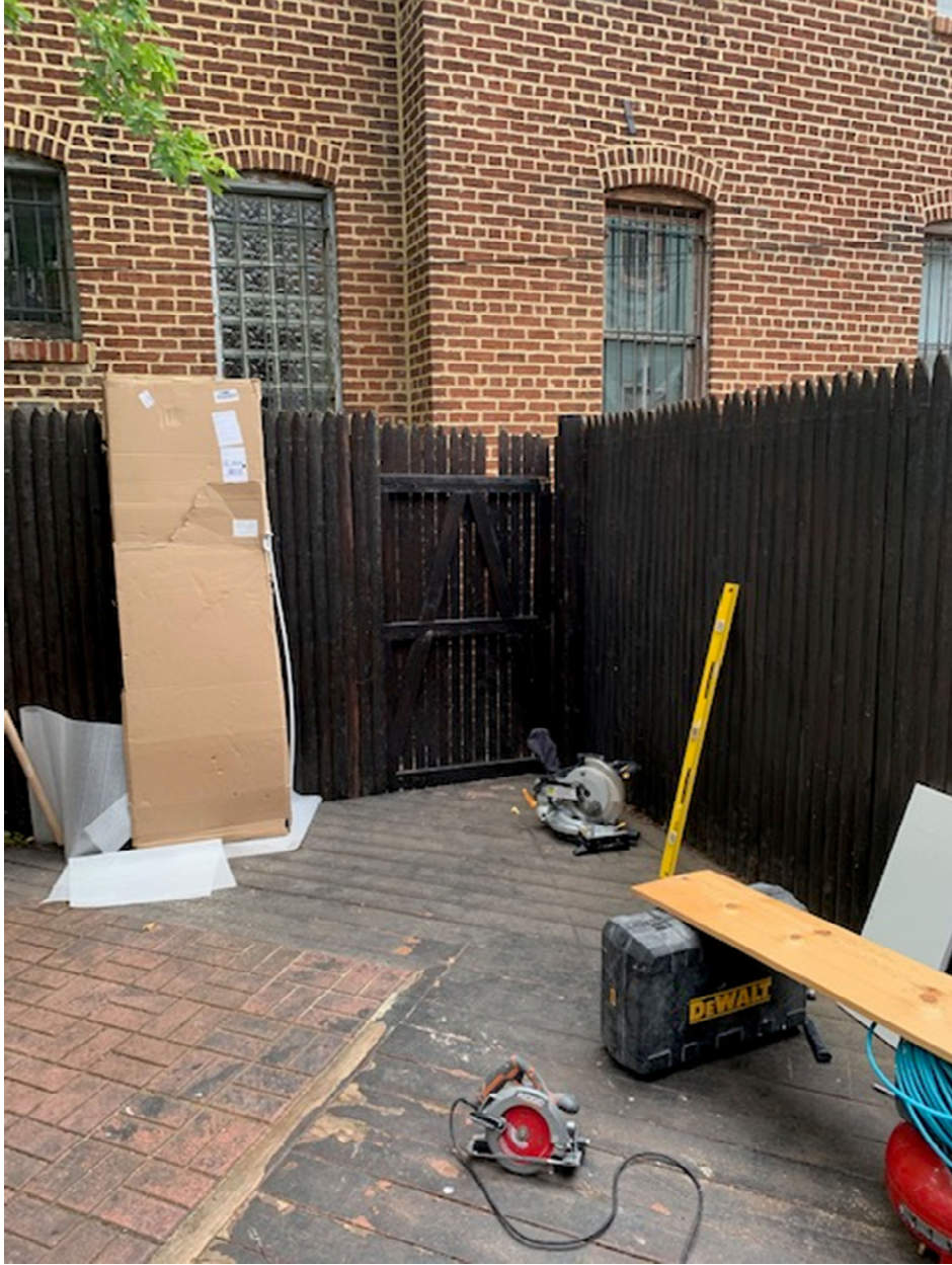
Interior View of 2205 Flager Fence
